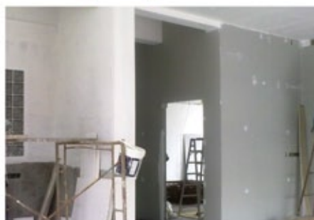
Downstairs learning centre partition.
